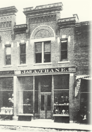
Trane Storefront La Crosse, Wisconsin 1891 Courtesy of the La Crosse (Wisconsin) Public Library Archives
